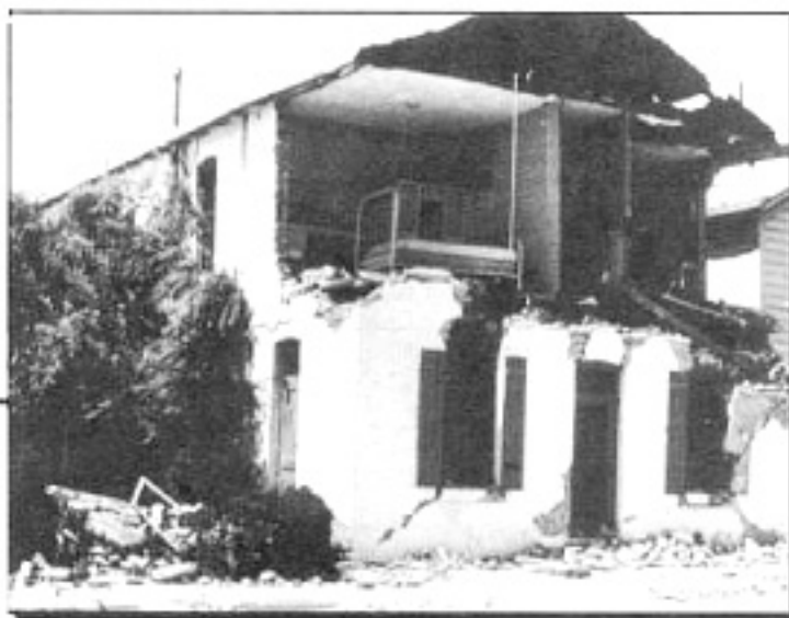
The plaster-covered brick walls of this building collapsed during a recent earthquake.
