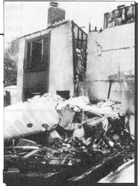
The unbraced water heater in this home fell during an earthquake; the resulting fire destroyed the home.
