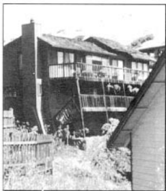
This hillside house was built on an unbraced tall wall that failed.
