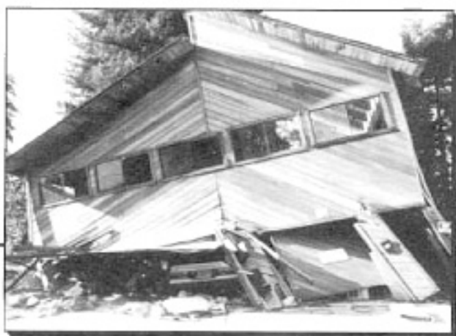
This mountain home was built over a garage, and its walls were not strong enough to withstand an earthquake.
