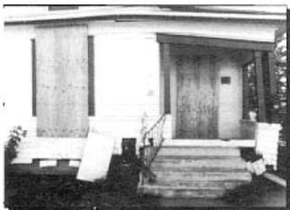
This home wasn't bolted and slid off its foundation.
