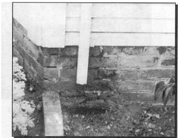
Note the bricks in an unreinforced masonry foundation.
