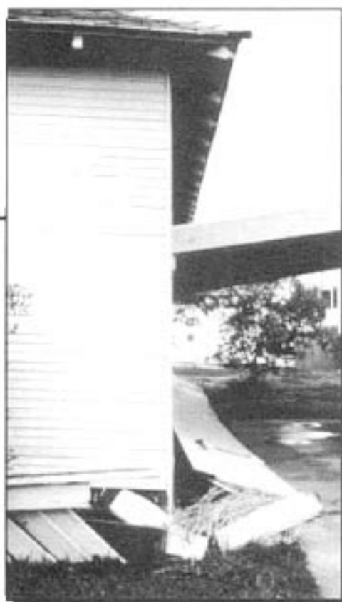
When this home's cripple wall failed, the building fell to the left, leaving behind on the ground the cripple wall from the side of the house.
