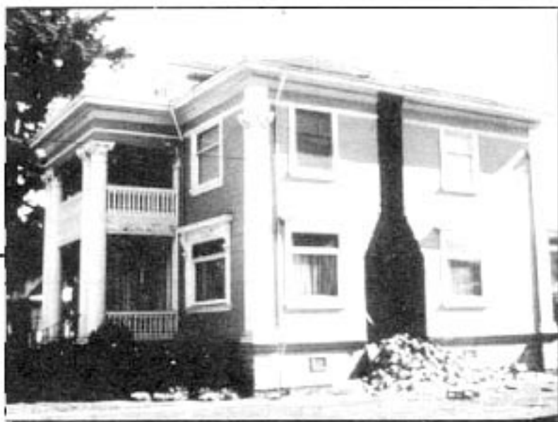
This unreinforced chimney fell during a recent earthquake.
