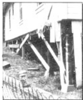
The pier-and-post foundation under this home shifted during a recent earthquake.
