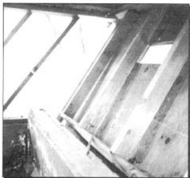
This photograph shows an interior detail of a home similar to the one at the left, showing substantial damage to a building with an unbraced tall wall.
